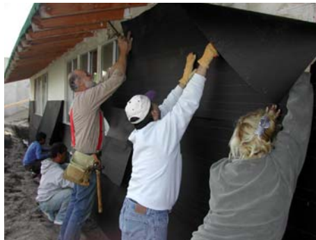
Part of the tar-wall team hard at work.
