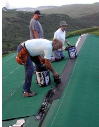
Almost done with the new roof.
