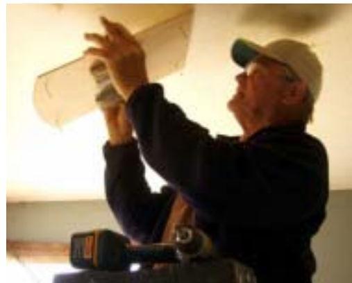
Installing the panel to receive the ceiling mounts.
